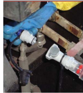
One connection waters all cells simultaneously
